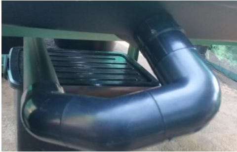
Return pipe attached to flow control outlet (2 x 45° elbows and 1 x 90° elbow)
